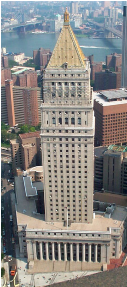
Aerial View of the Courthouse
