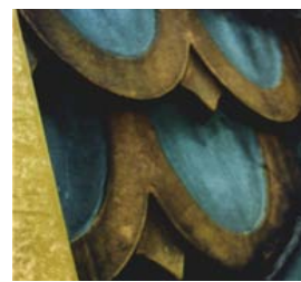
Detail of glazed terra-cotta roof tiles.
